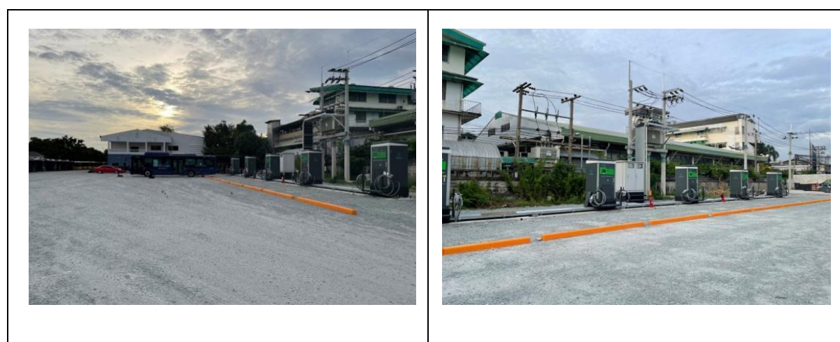
Figure 3: Example pictures of bus station in PoA 02 ‘Phra Pradaeng E-bus station and the charging station’
